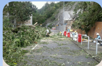
The project team was removing broken branches and refuse at Hiu Ming Street heading to CCC Mong Man Wai College
