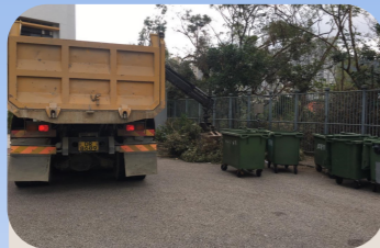
The project team was removing broken branches and refuse at HKSKH Bishop Hall Secondary School after typhoon
