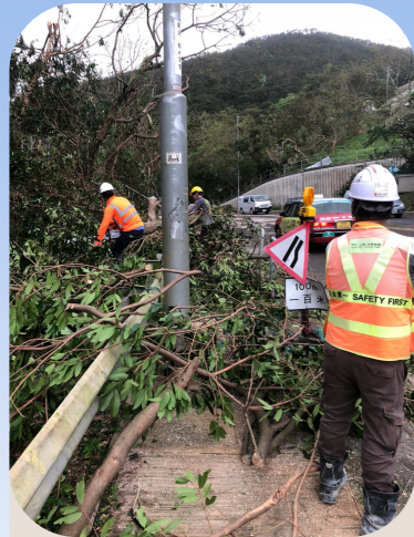
The project team was removing fallen trees blocked at Ma Yau Tong
